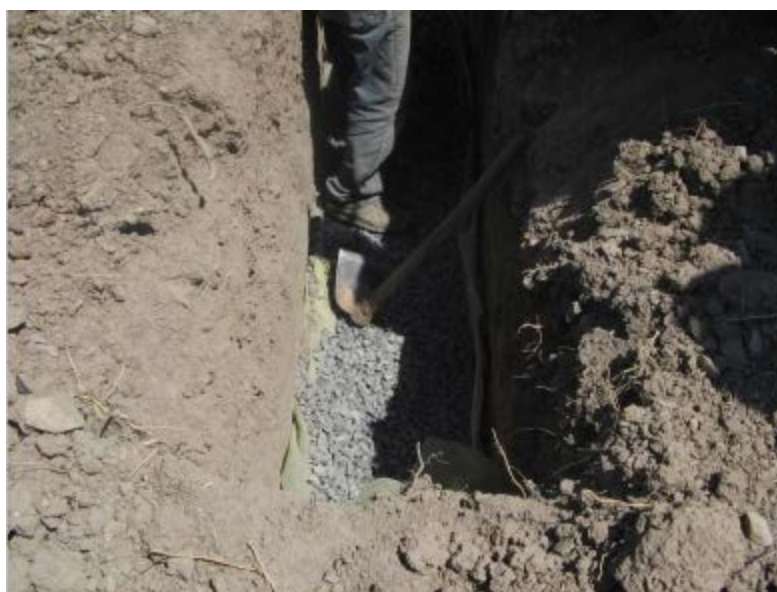
Fig. 6. Pockets in buried stones (in phase of realization)
